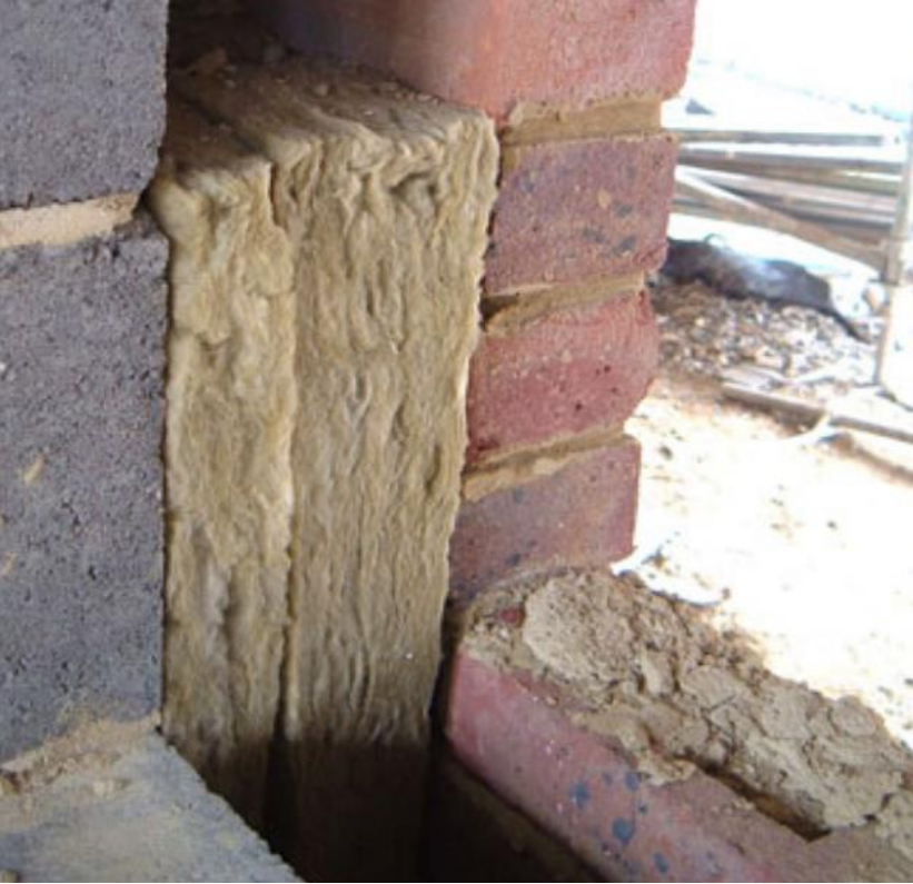
Cavity Wall insulation
