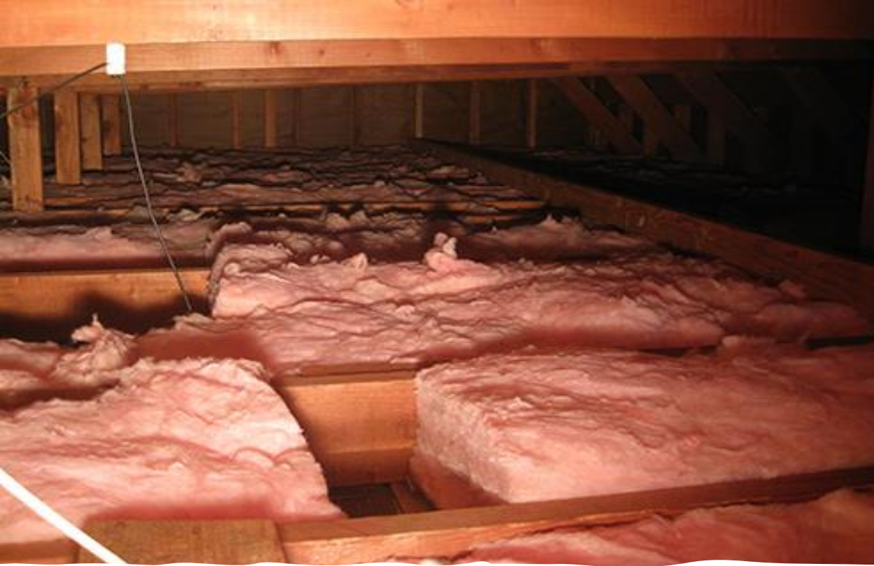
Roof and loft insulation
