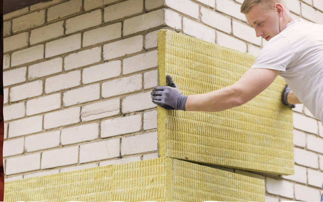
Solid wall insulation
